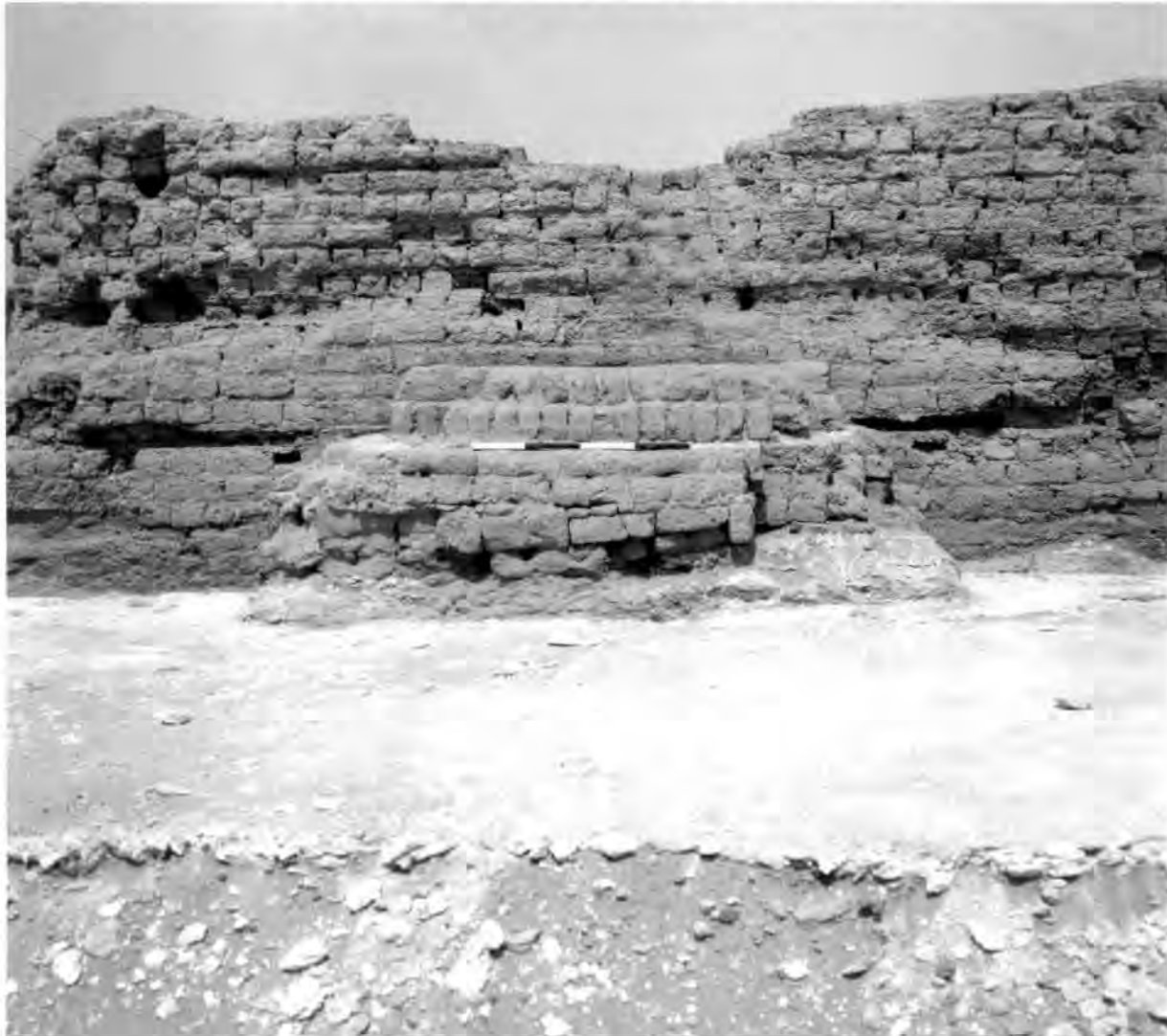
Figure 6.15. The south face of the north pylon tower, viewed to the north, showing the brick nib with the outline of a ramp preserved as an angled course of brickwork towards the bottom. In the foreground is the gypsum surface [3414] of the central platform.
