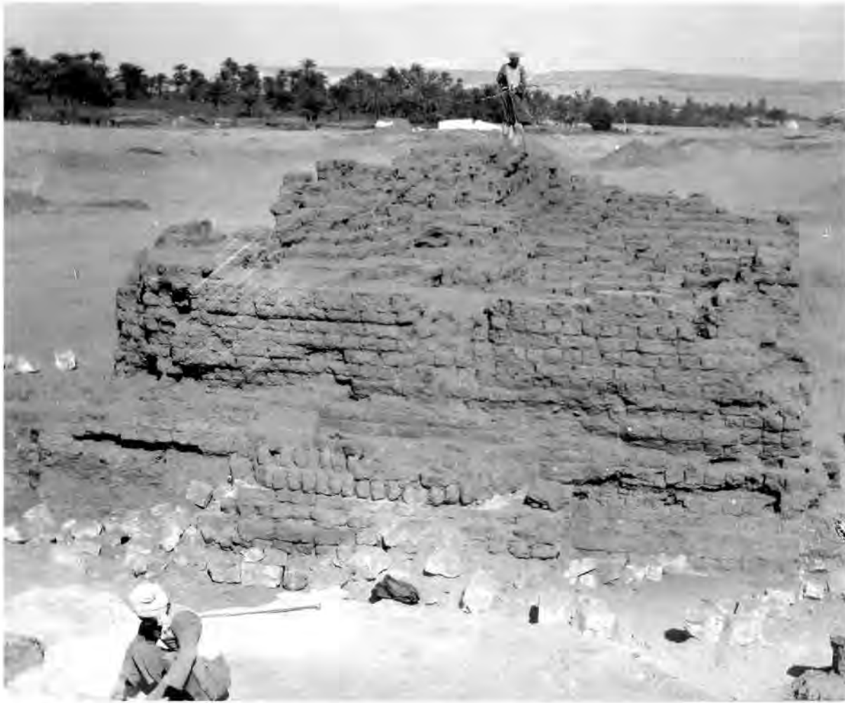
Figure 6.16. The gateway of the First Pylon during excavation in 1931, viewed to the north. Note the limestone blocks remaining from the platform, scarcely any of them, it would seem, in situ . Archive photograph 31/32.A127.
