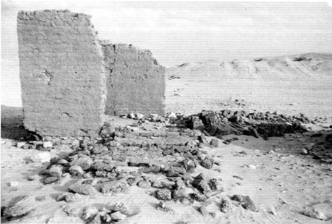
Figure 4.4. A modern example of sheet collapse, at abandoned huts west of the South Tombs at Amama.
