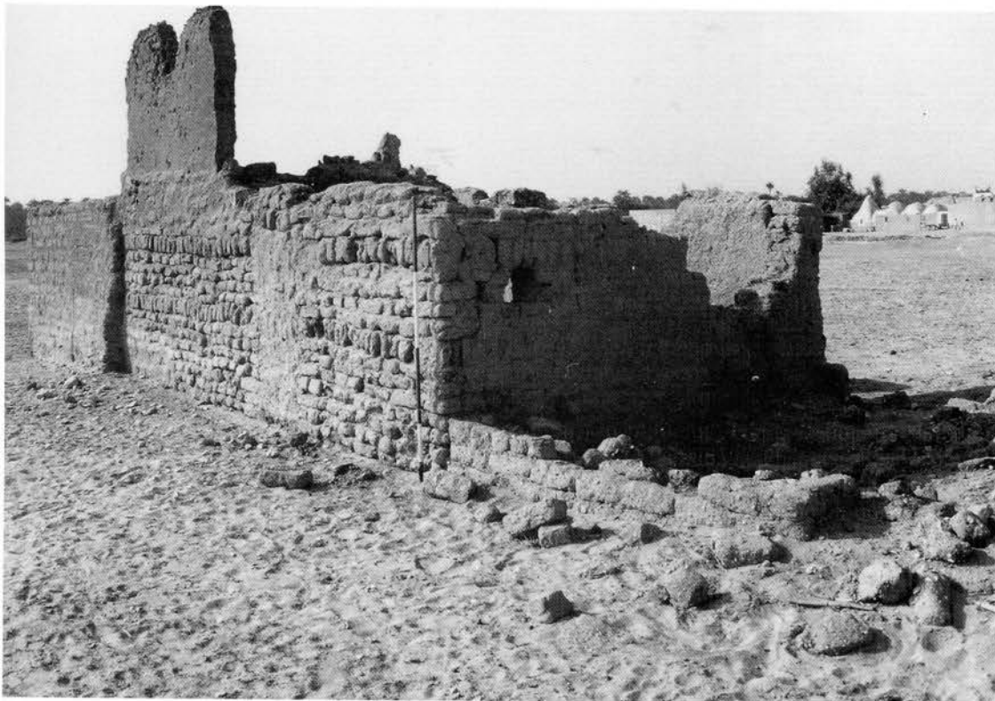
Figure 4.1. The “experimental house” at Amarna, photographed in 1992 from the south-east.
