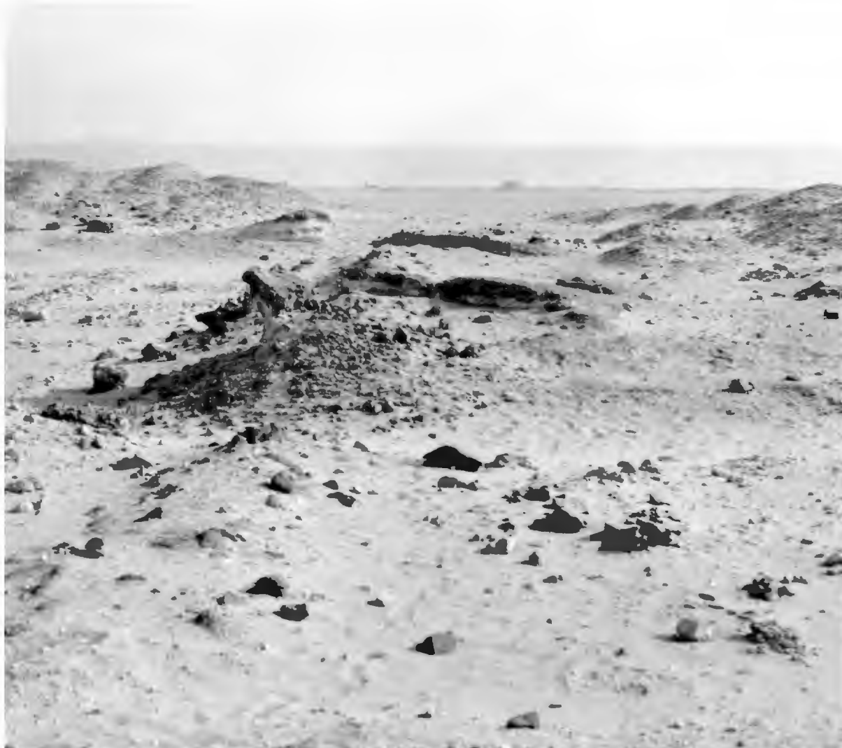
Figure 8.2. Remains of the embankment along the rear of the Sanctuary, looking north.
