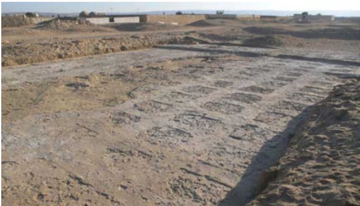
Figure 4. The gypsum concrete foundation platform at the end of the cleaning, viewed to the east.
