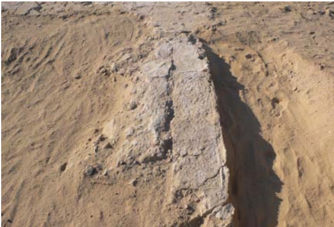
Figure 9. Foundations for a threshold at the western end of the cleared area of the first court, viewed to the south.
