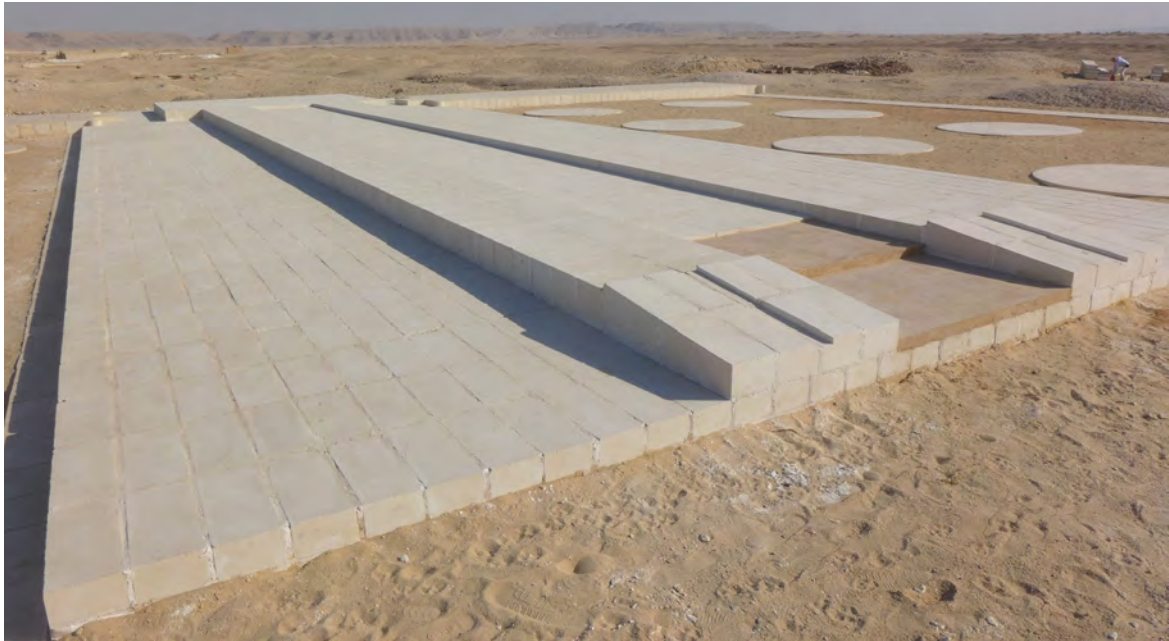
Figure 14. The beginning of the staircase that led to the offering-platform at the front of the Great Aten Temple. The slots in the surface of the sloping limestone blocks are awaiting red granite inserts. View to the south-east. Photo by B. Kemp.
