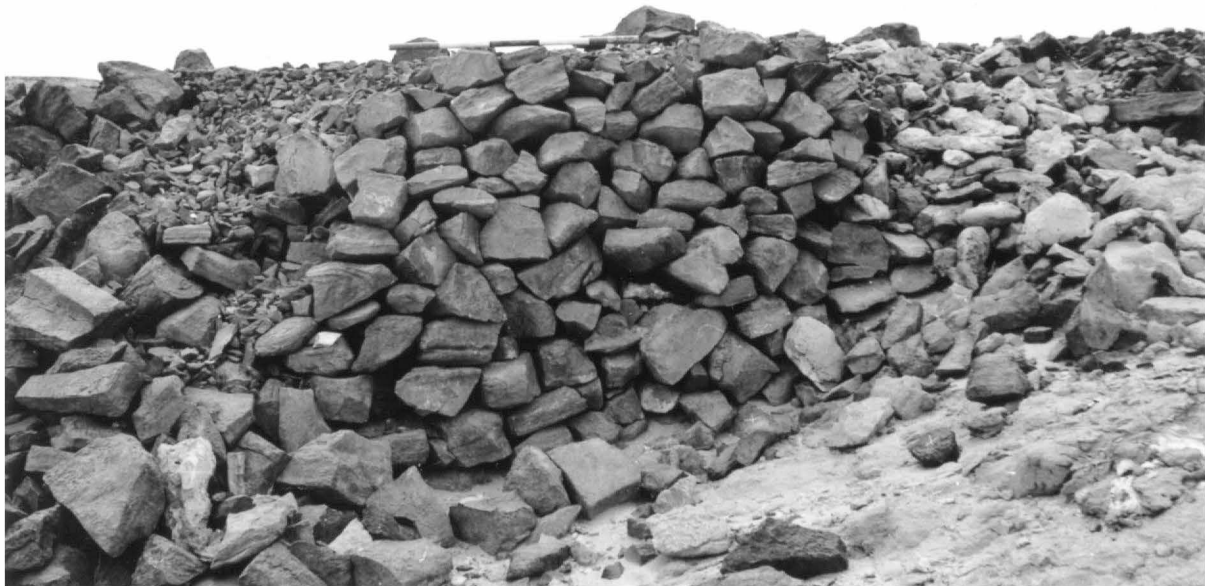
Figure 13.3: Detail of the main quarry road: two views of the embankment near quarry P.
